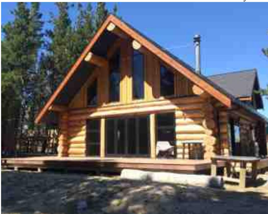
*Orientation, openings and overhangs: note how the upper windows are shaded by the overhangs. Johnson house - Log Building Course Tour*
