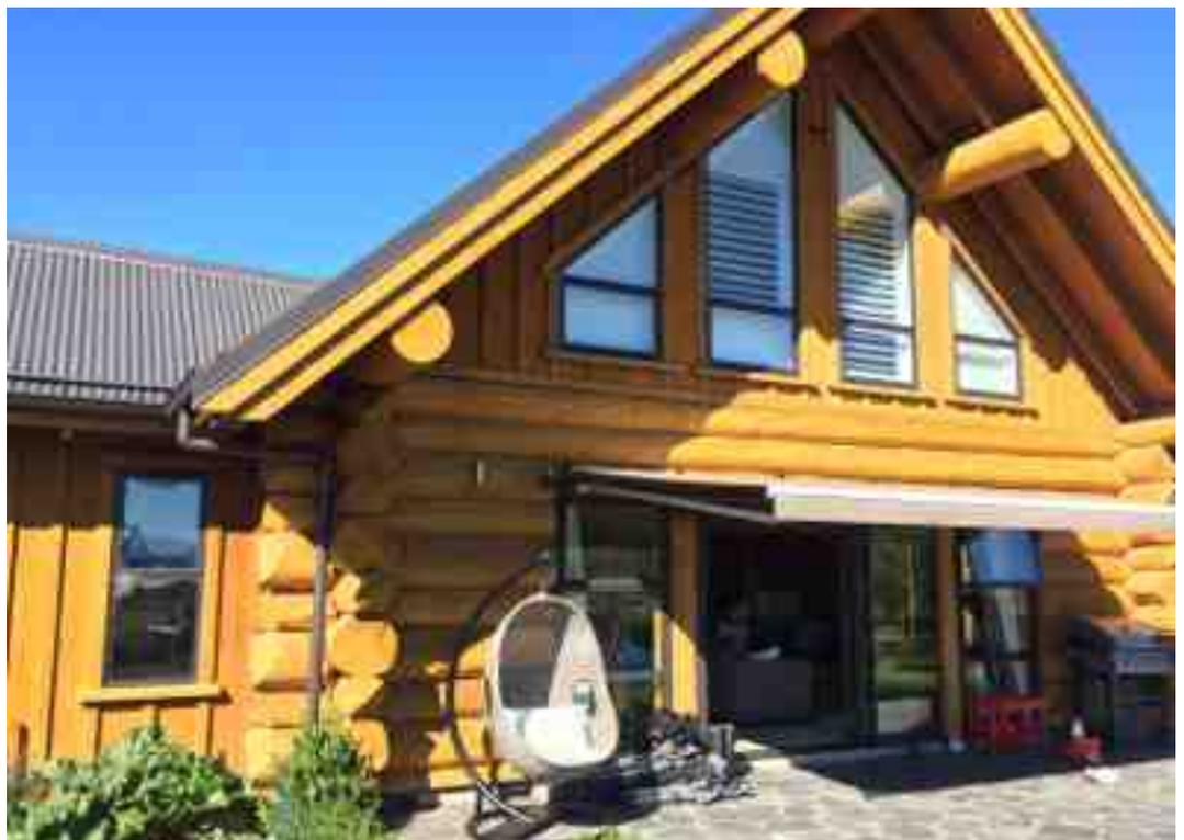
*The framed walls incorporated in this log house will need insulation installed. - Log Building Course Tour*
